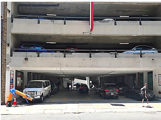
180 Car attached parking garage
