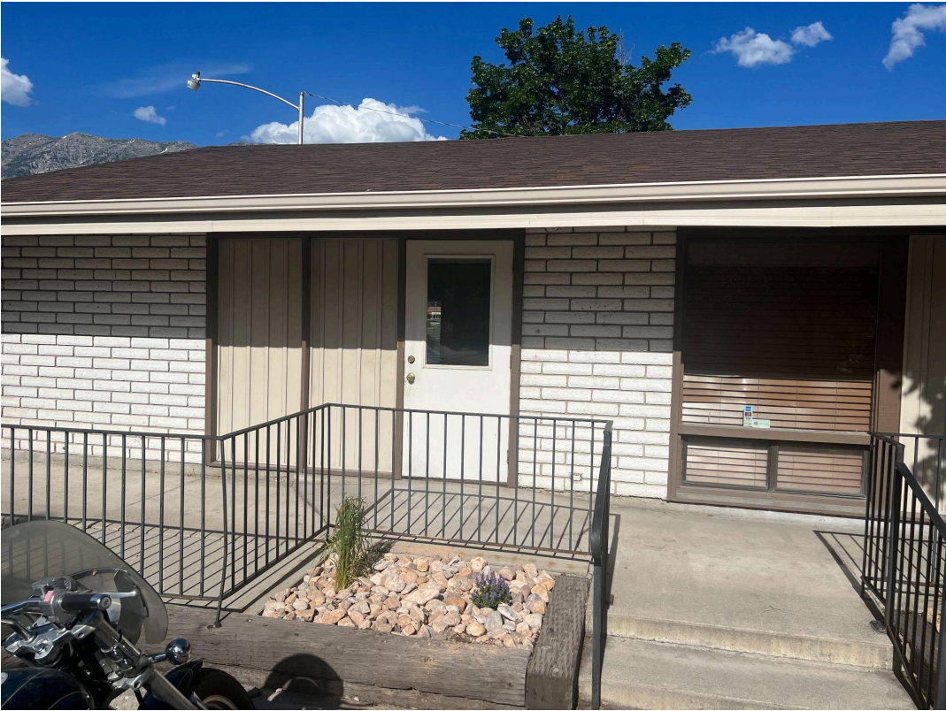
Front View - from the parking lot
