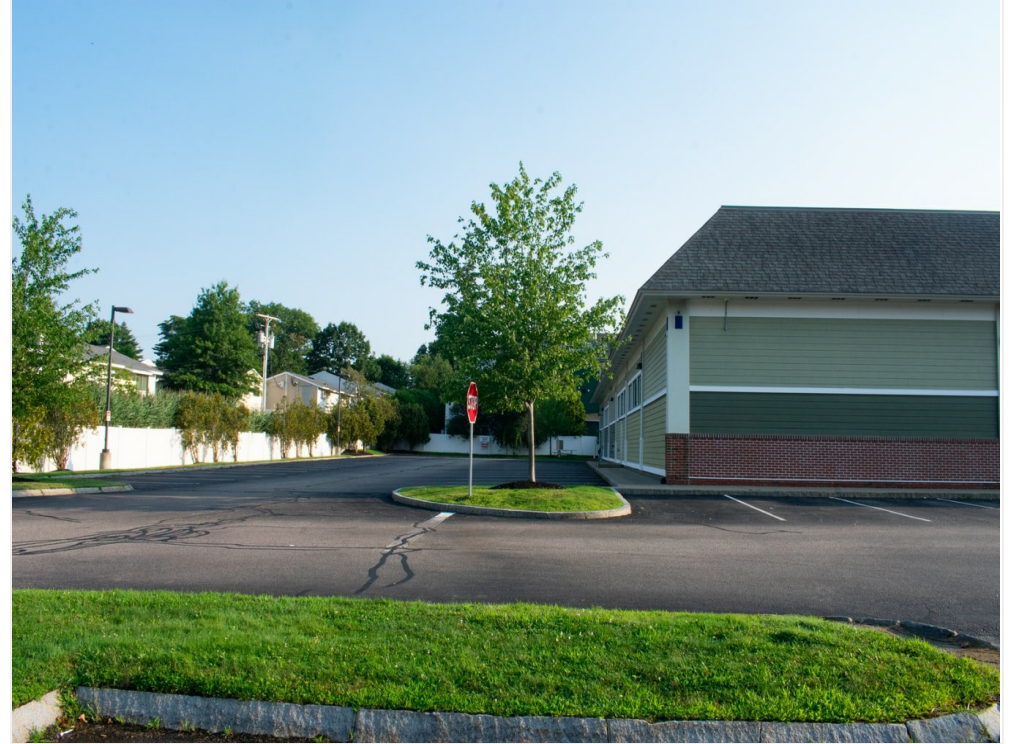
Back of building
