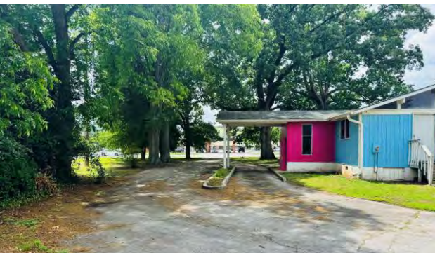
Former Drive Thru
