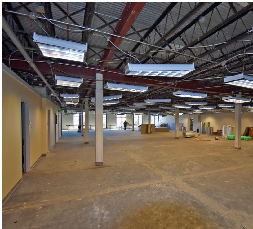
3rd Floor interior
