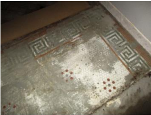
Existing flooring boarder
