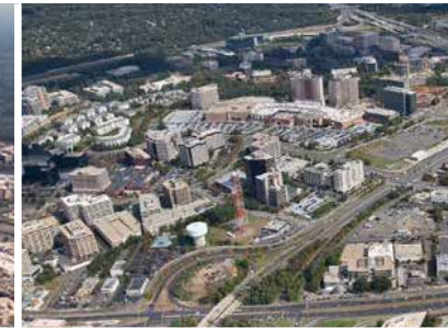
Delivery of the $2.75B Silver Line Metrorail service and $1.4B Express Lanes (Capital Beltway) create a multi-dynamic infrastructure platform providing the ability to transform Tyson's into a 24/7 urban center
