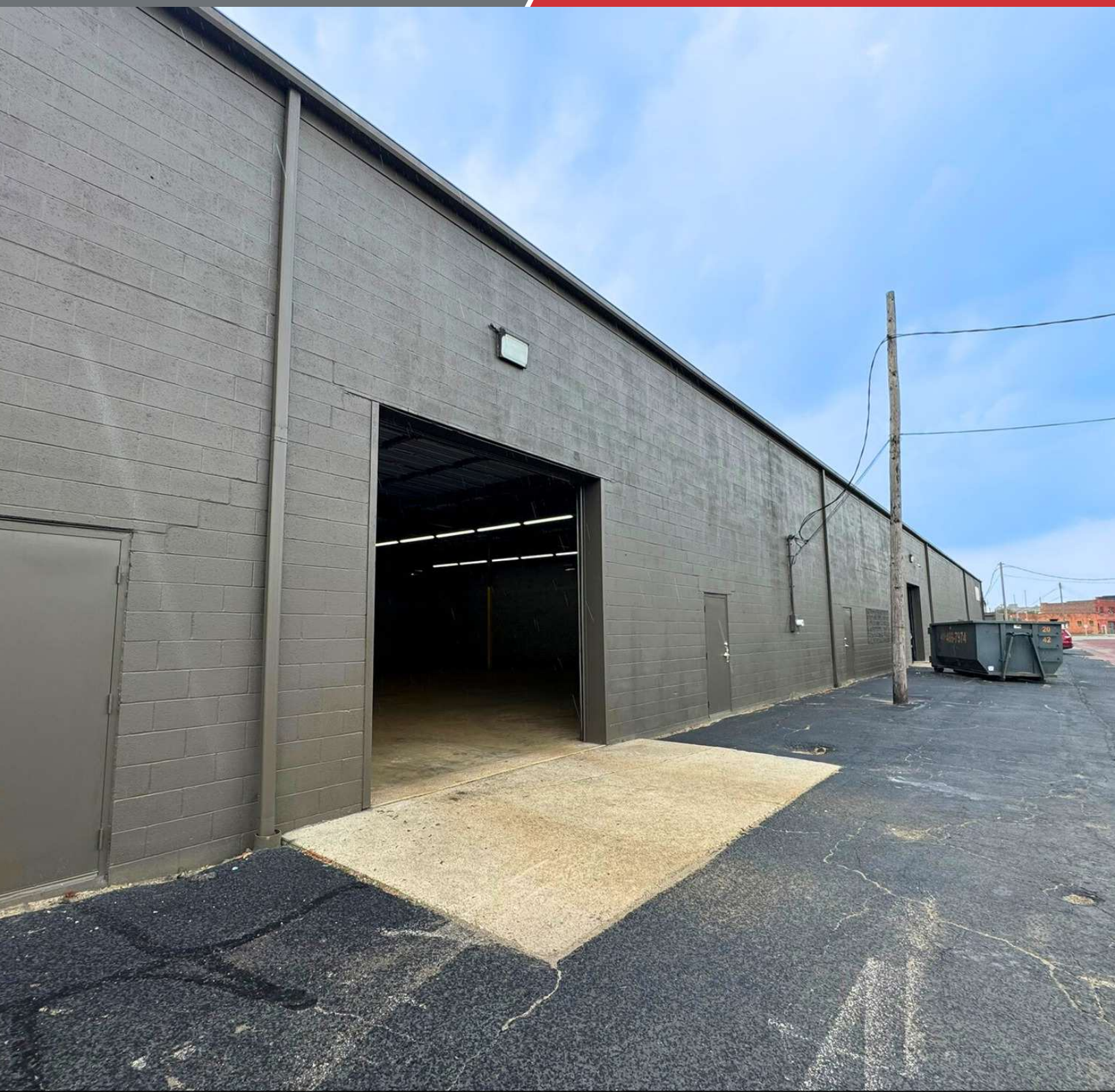
Newer Pavement, Fresh Paint On Exterior, And New Roof
