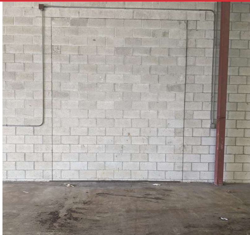
Knock Out Connecting Adjacent Bay
