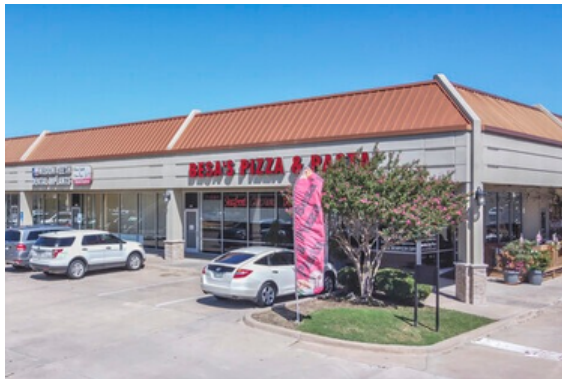
14856 PRESTON ROAD BUILDING 1
