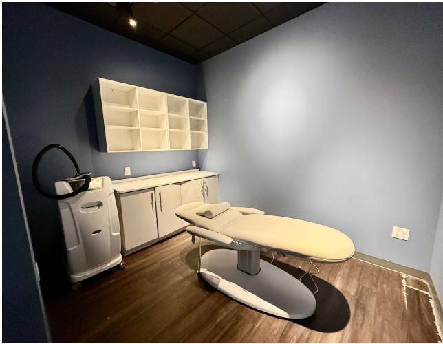
Private treatment room. Casework, lighting and finishes remain; the cryotherapy and treatment beds shown will be removed.
