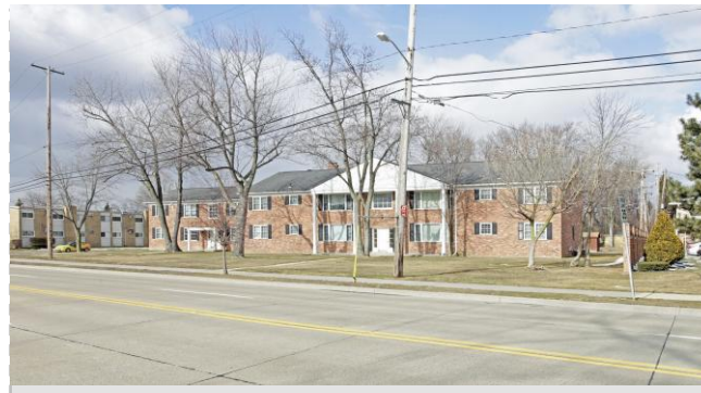
JEFFERSON AVE APARTMENTS
