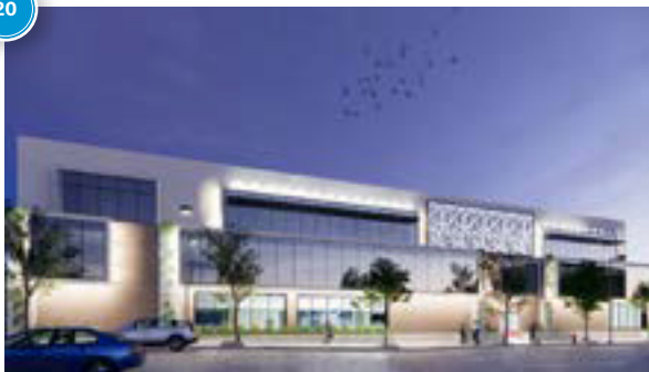
Aegis at ParkPointe 17017 W Ventura Blvd
