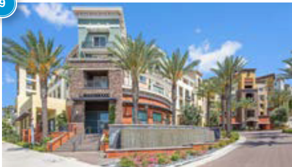
The Boulevard Apartment Homes 20600 Ventura Blvd
