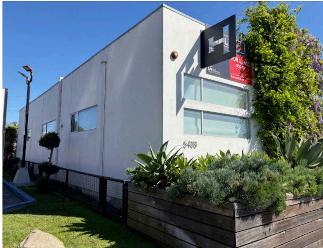
8 Ft tall private, locked yard
