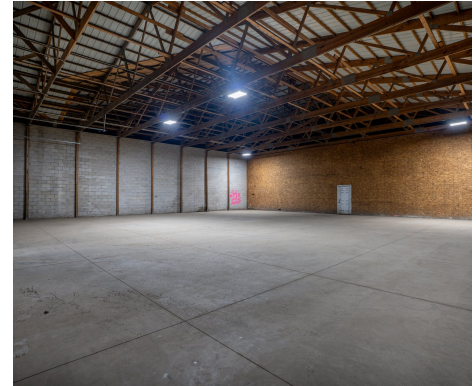
Unit B – cold storage
