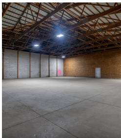
Unit B cold storage
