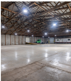
Unit A clear-span
