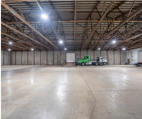
Unit A – ±26,600 SF clear-span
