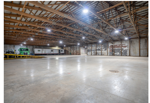
New LED throughout Unit A
