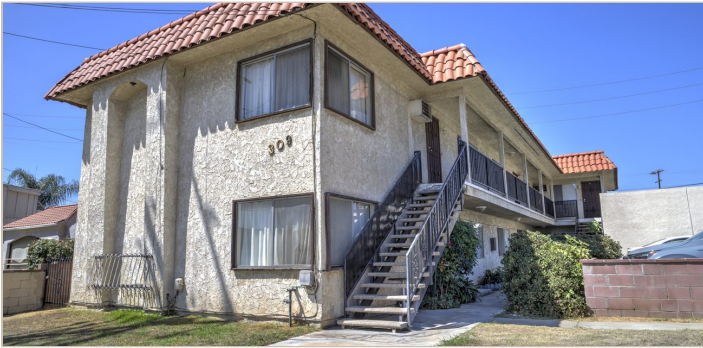
Building front. Six units over two levels, tile and flat roof, exterior stair to the upper walkway.
