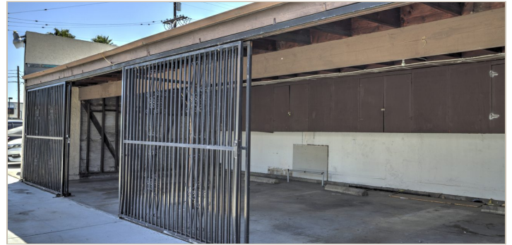
Six enclosed garages behind a gated entry, with individual tenant storage cabinets along the rear wall.
