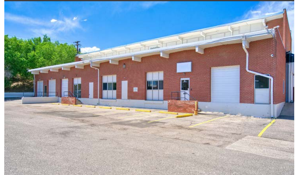
2590 WEST 2ND AVENUE, UNITS 24 & 25
