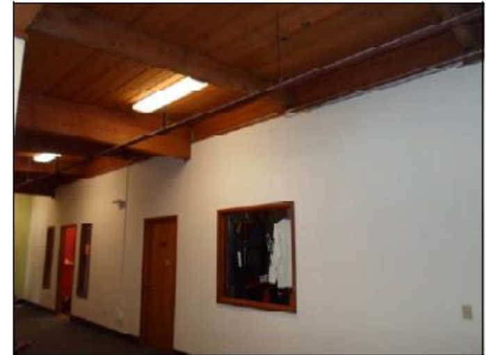
Another second floor hallway photo
