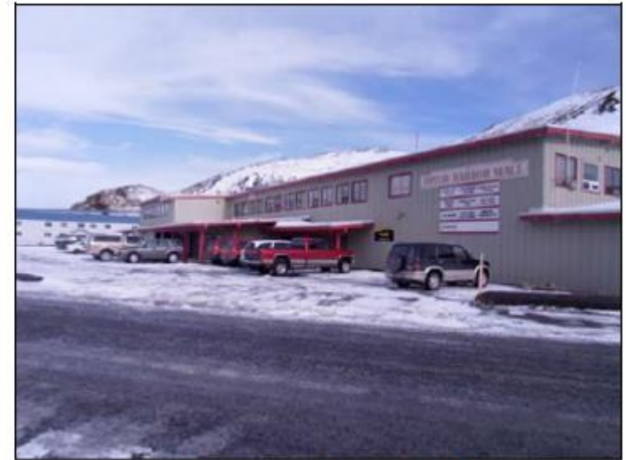
Northeast view of front of building
