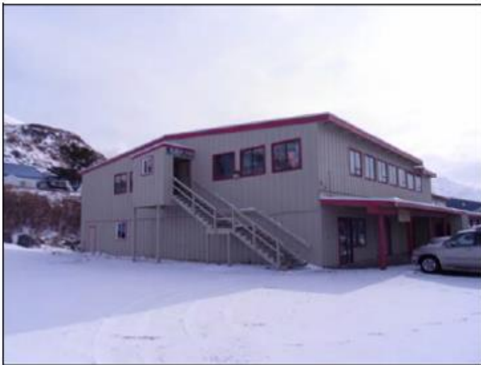
Southeast view of north side of subject
