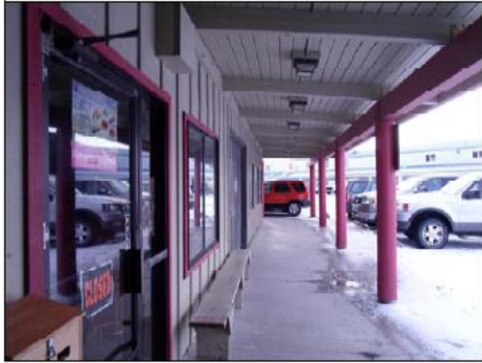
First floor exterior walkway
