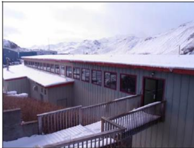
Back side of property
