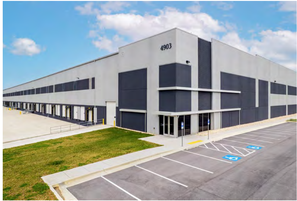
Building A | 365,400 sf | 4903 Winchester Avenue
