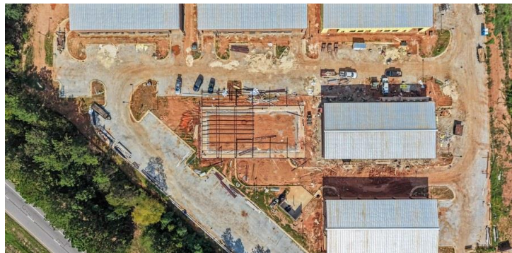
Phase 2 building pod, overhead
