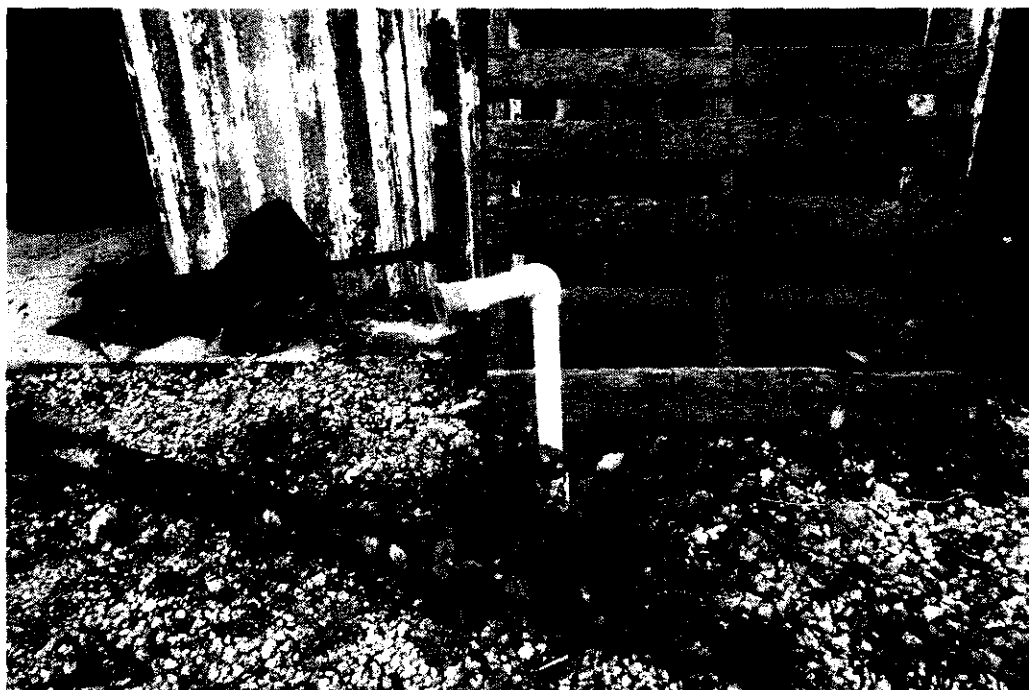
View of the on-site water supply well.
