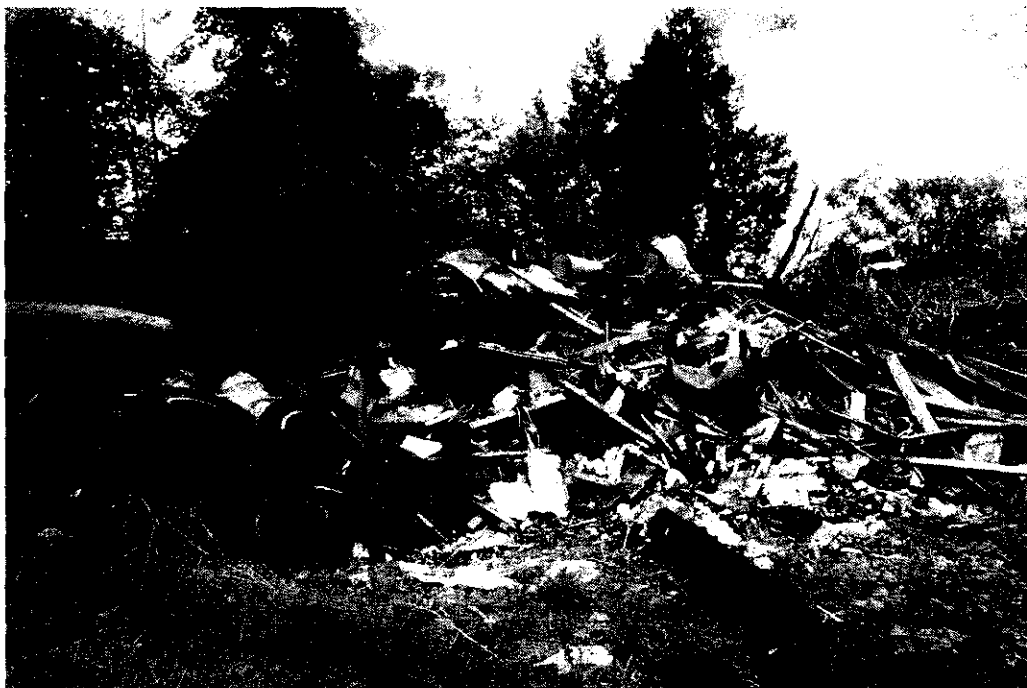
View of one of the piles of debris located along the eastern property boundary of the subject site facing east.
