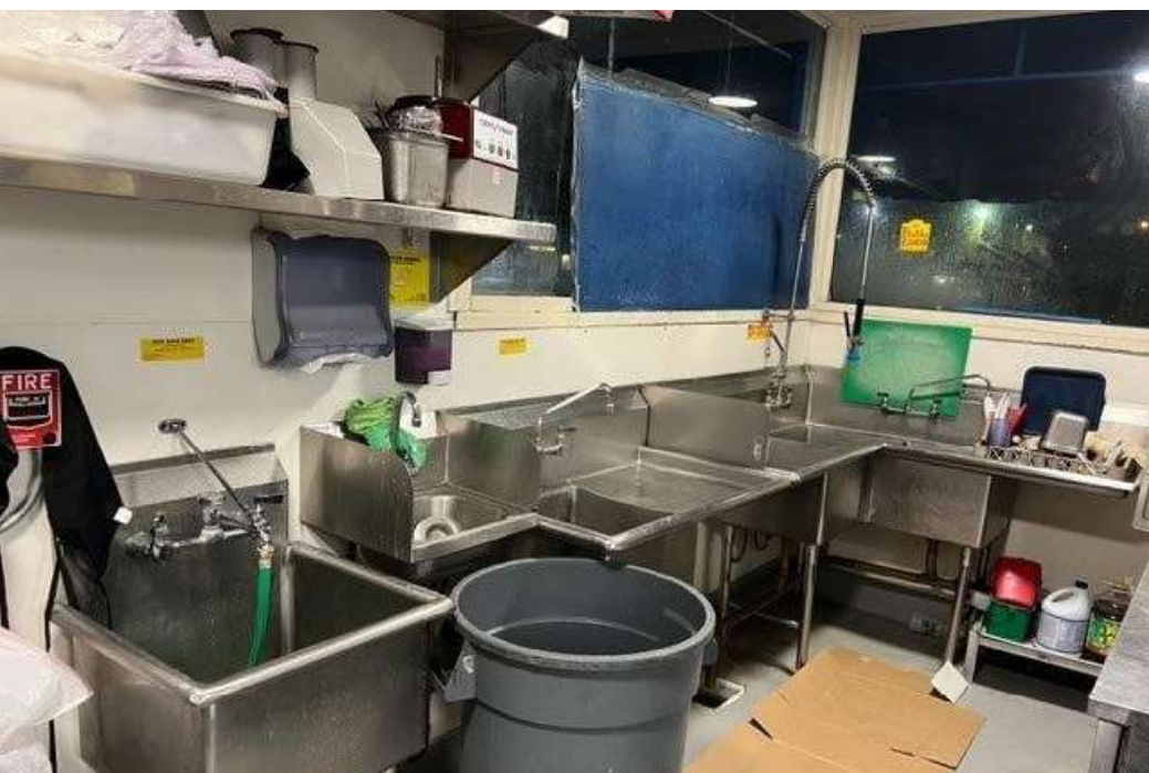
Dishwashing Area , Mop & Hand Wash Sink
