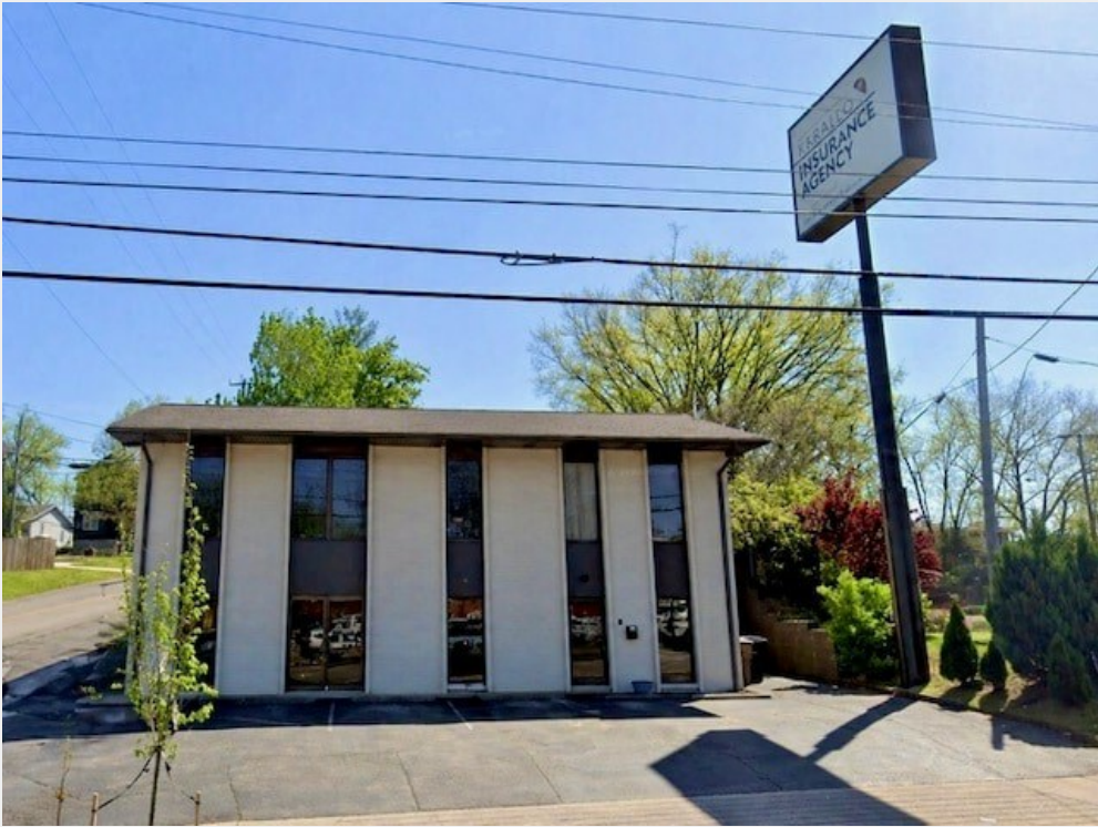
296 White Bridge Pike
