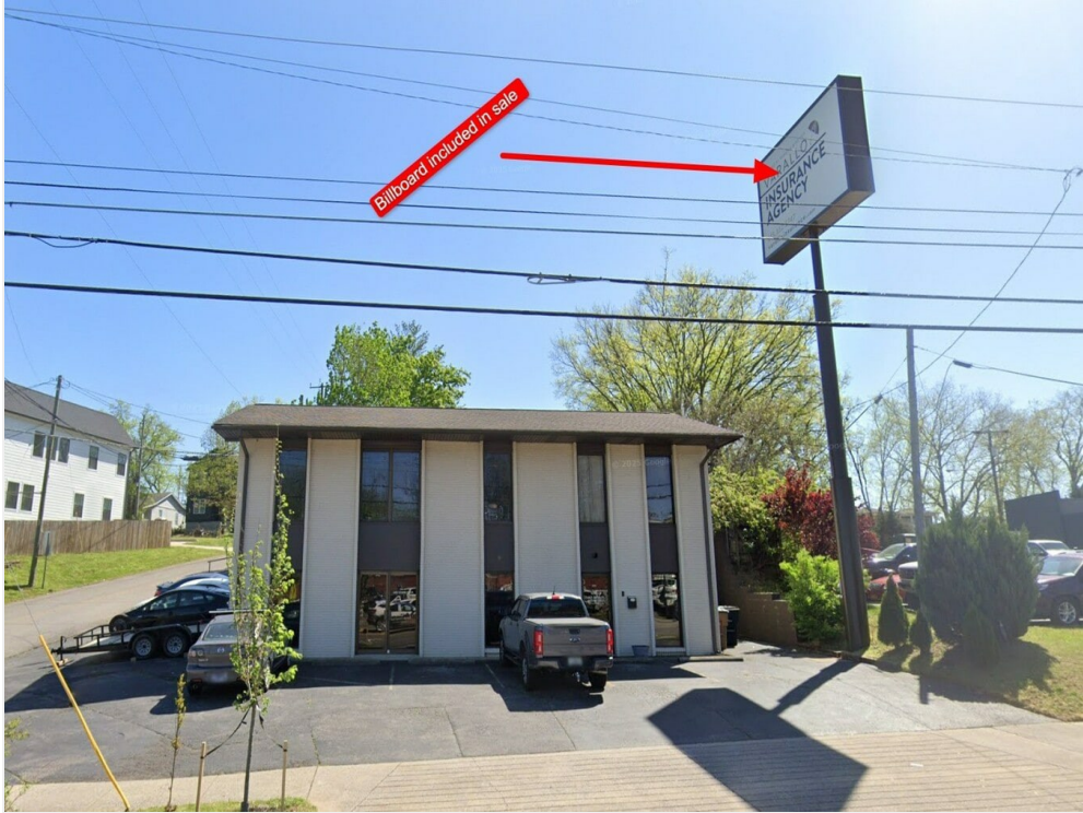
296 White Bridge Pike
