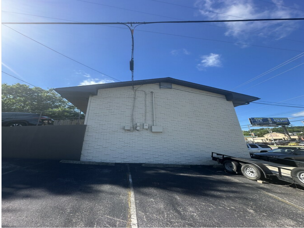
296 White Bridge Pike
