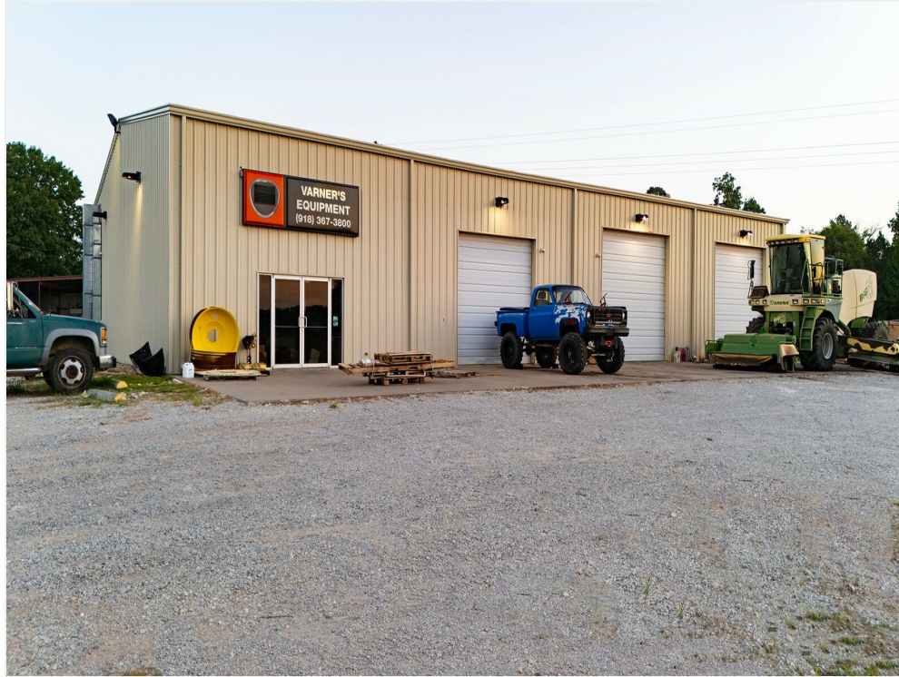
Front of Building
