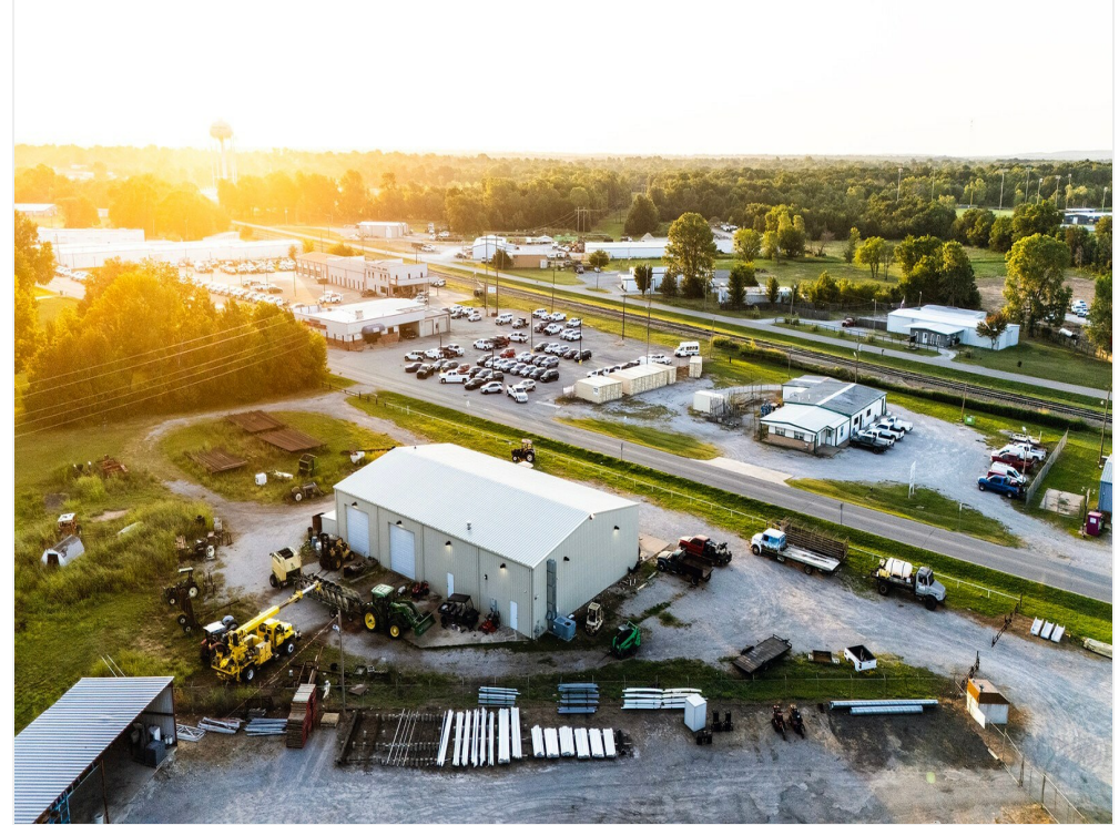
View of Exterior Wash Bay
