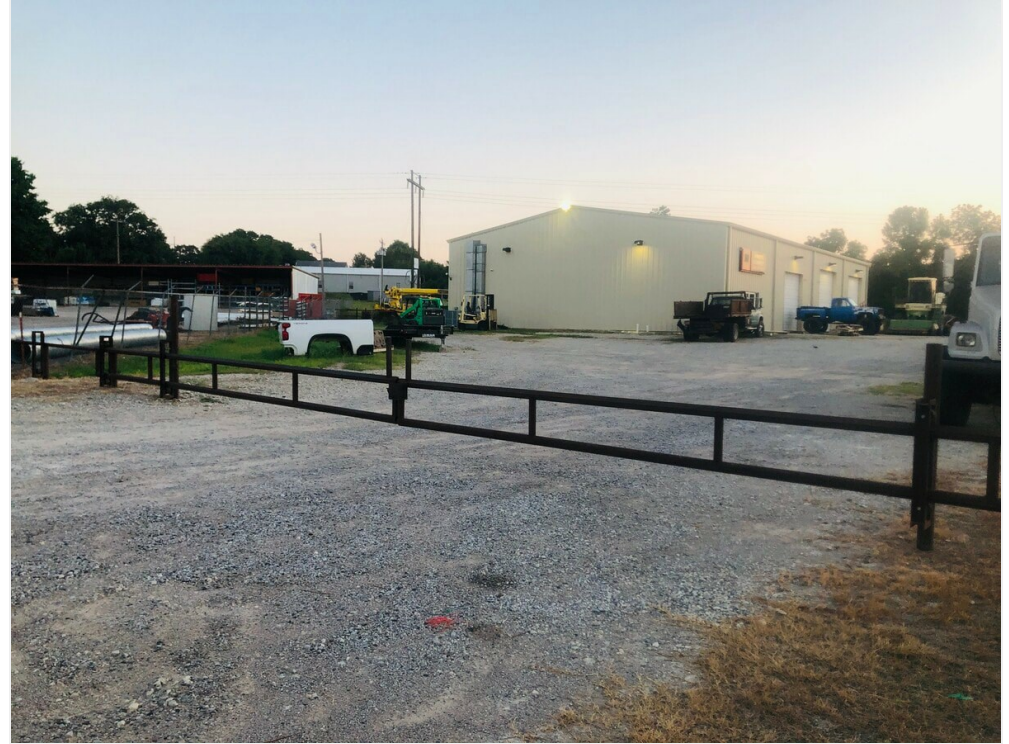
Private Entry Gate
