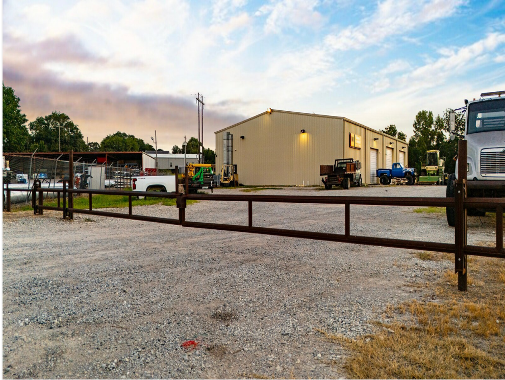
View of West Side
