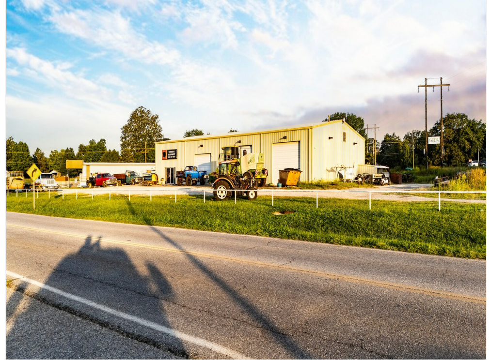
Building of East Facade
