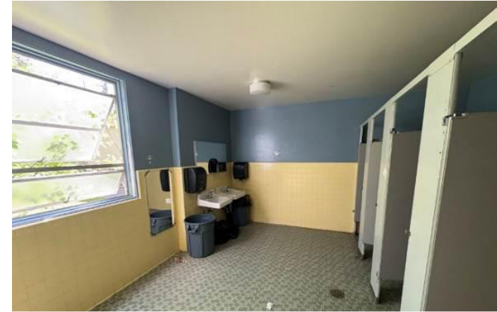
MAIN BUILDING - RESTROOM
