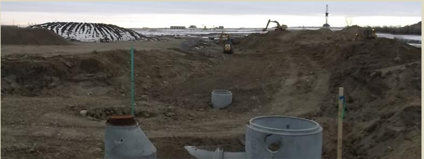
Jan 02 – 11 th Ave. Backfill/Compaction Sanitary run between manholes
