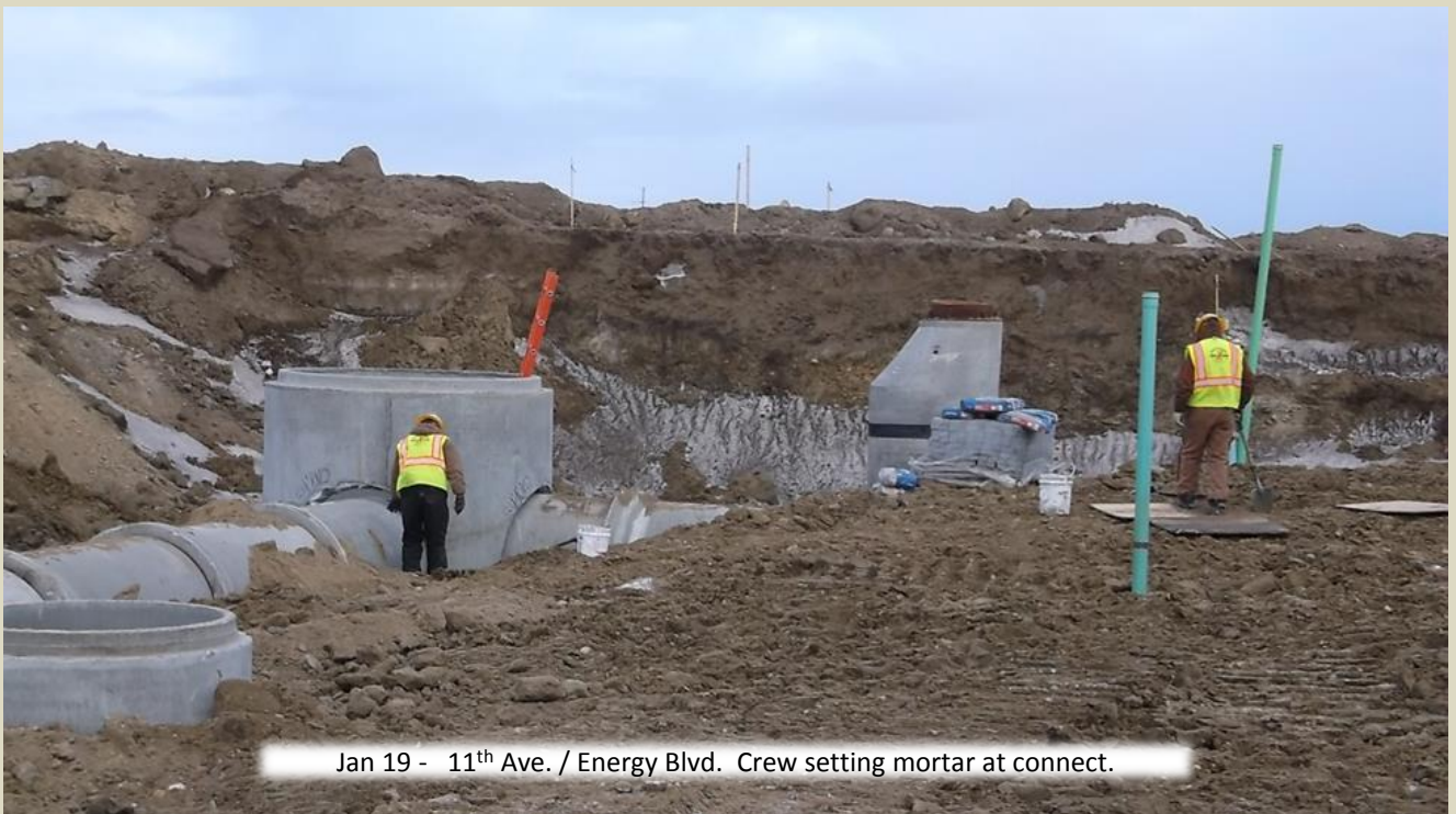
Jan 19 - 11 th Ave. 36" RCP run north
