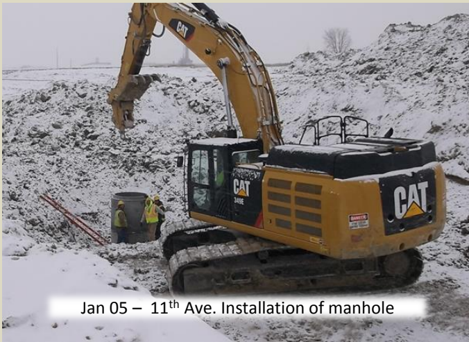
Jan 02 – 11 th Ave. Sanitary Crew installing PVC and manhole
