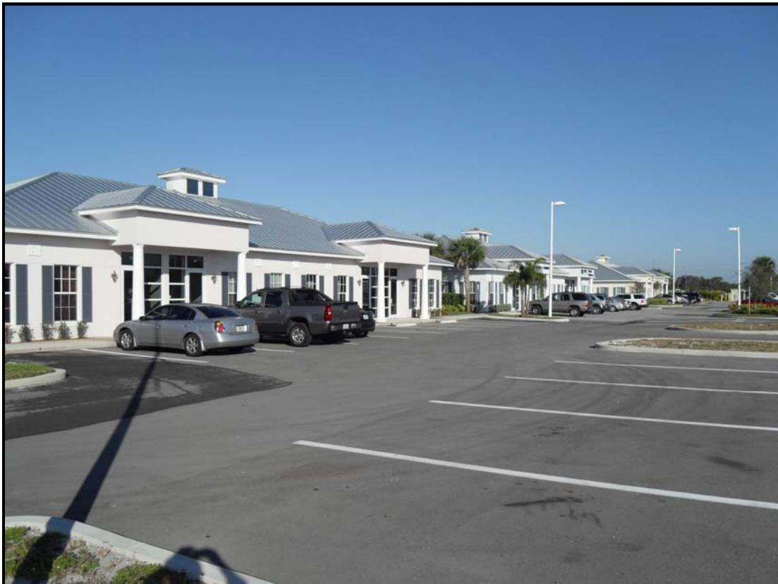
LOOKING NORTH AT EXISTING BUILDINGS #2, #3 AND #4
