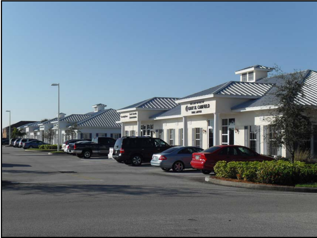
LOOKING SOUTH AT EXISTING BUILDING #2, #3 AND #4
