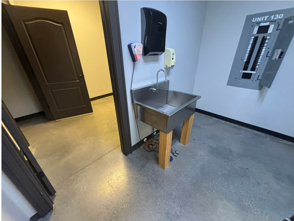
Sinks in room
