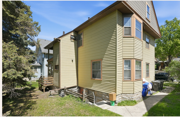
Rear stairwell to basement unit
