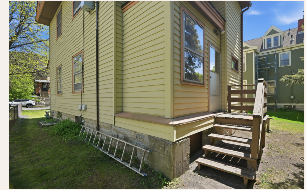
Rear stairs to unit 1
