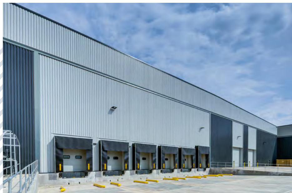
5 dock level doors & 1 euro dock level door
