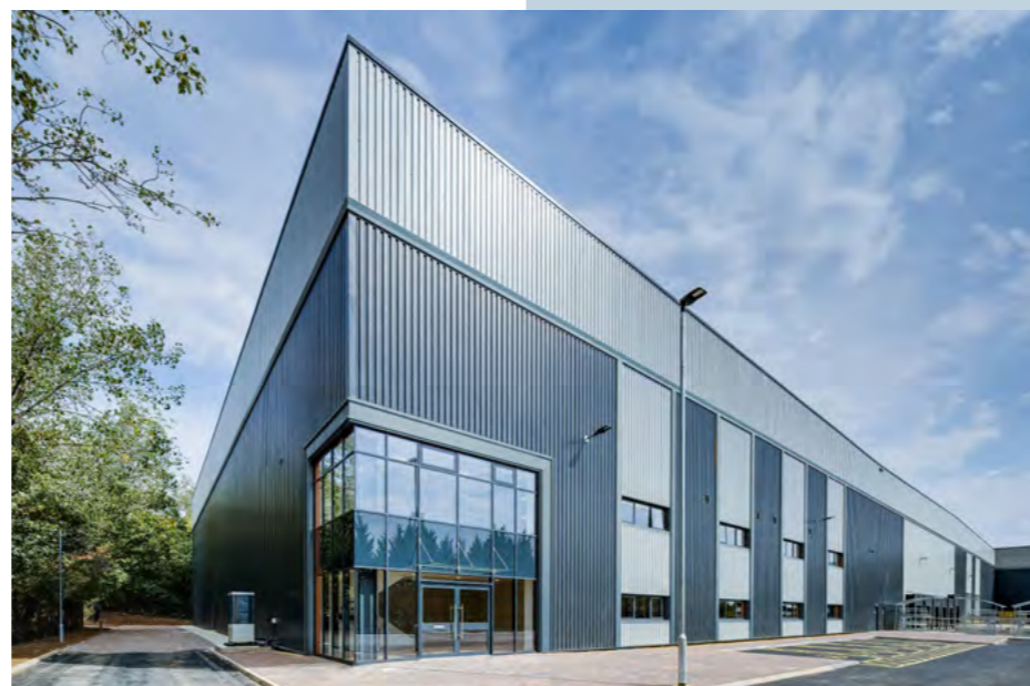
Reception entrance & EV charging unit
