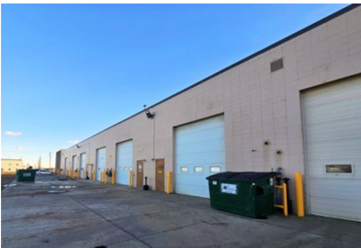
8 x 12 x 14' Overhead Doors + 2 x 16 x 16' Overhead Doors
