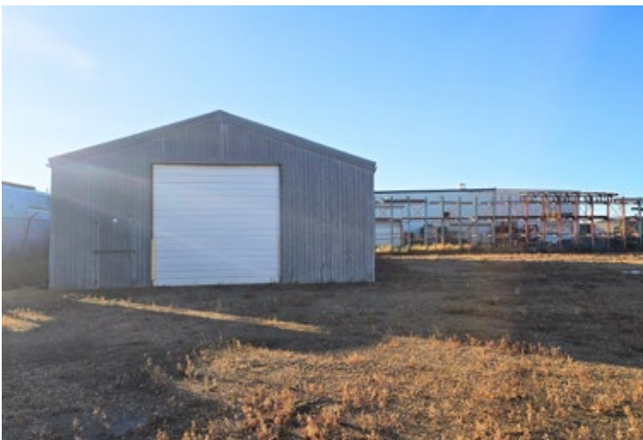
Metal Siding Building 2,400 SF (30x80')
