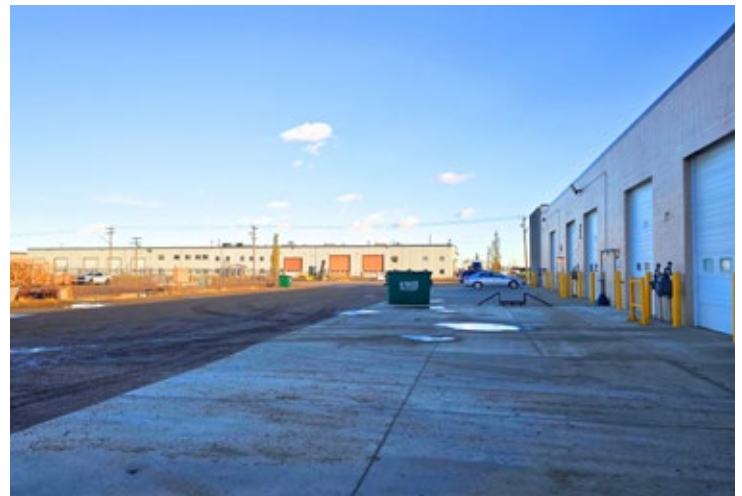
Concrete Apron with Large Marshalling Area
