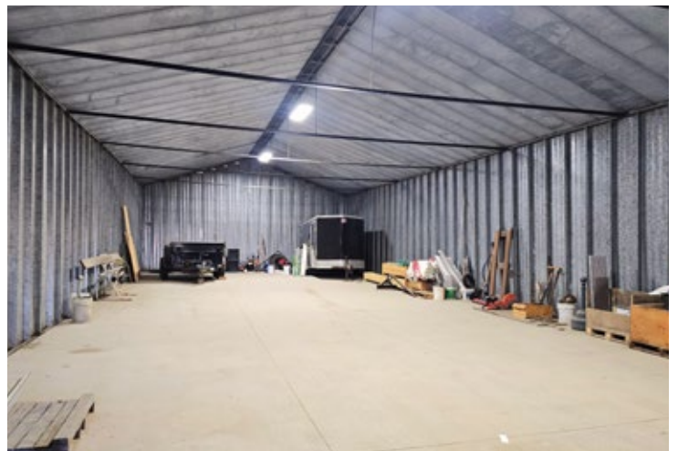
Wired w/Electrical, Cement Poured Floor
