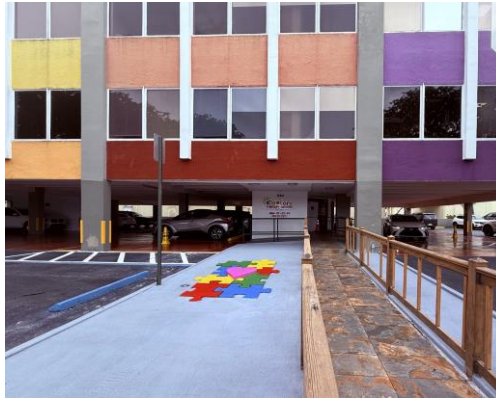
ACCESSIBLE RAMP & WALKWAY
