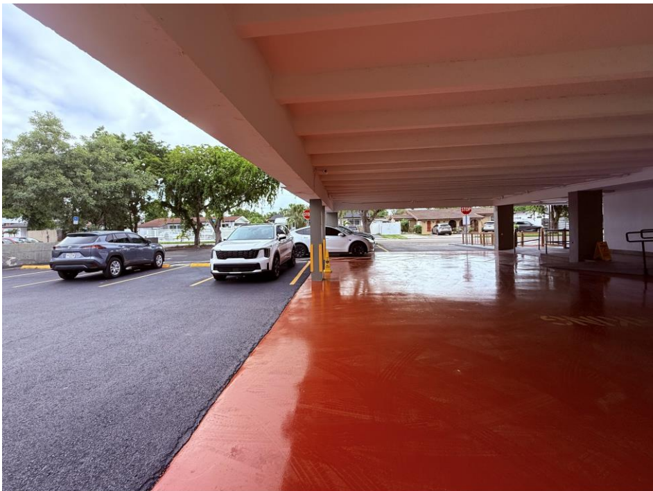
COVERED DRIVE & LOADING AREA
