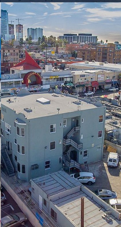
Alvarado Apartments - Westlake
