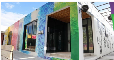
The Campus on 5th 35,000 SF Big Move Properties
