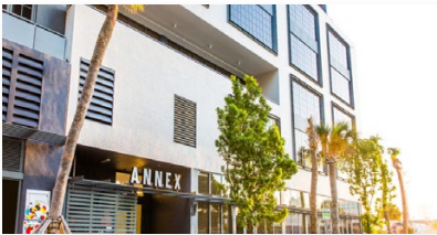
The Annex 60,000 SF Brick & Timber
