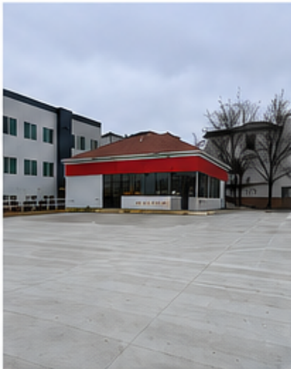
AMPLE PARKING & ACCESS
