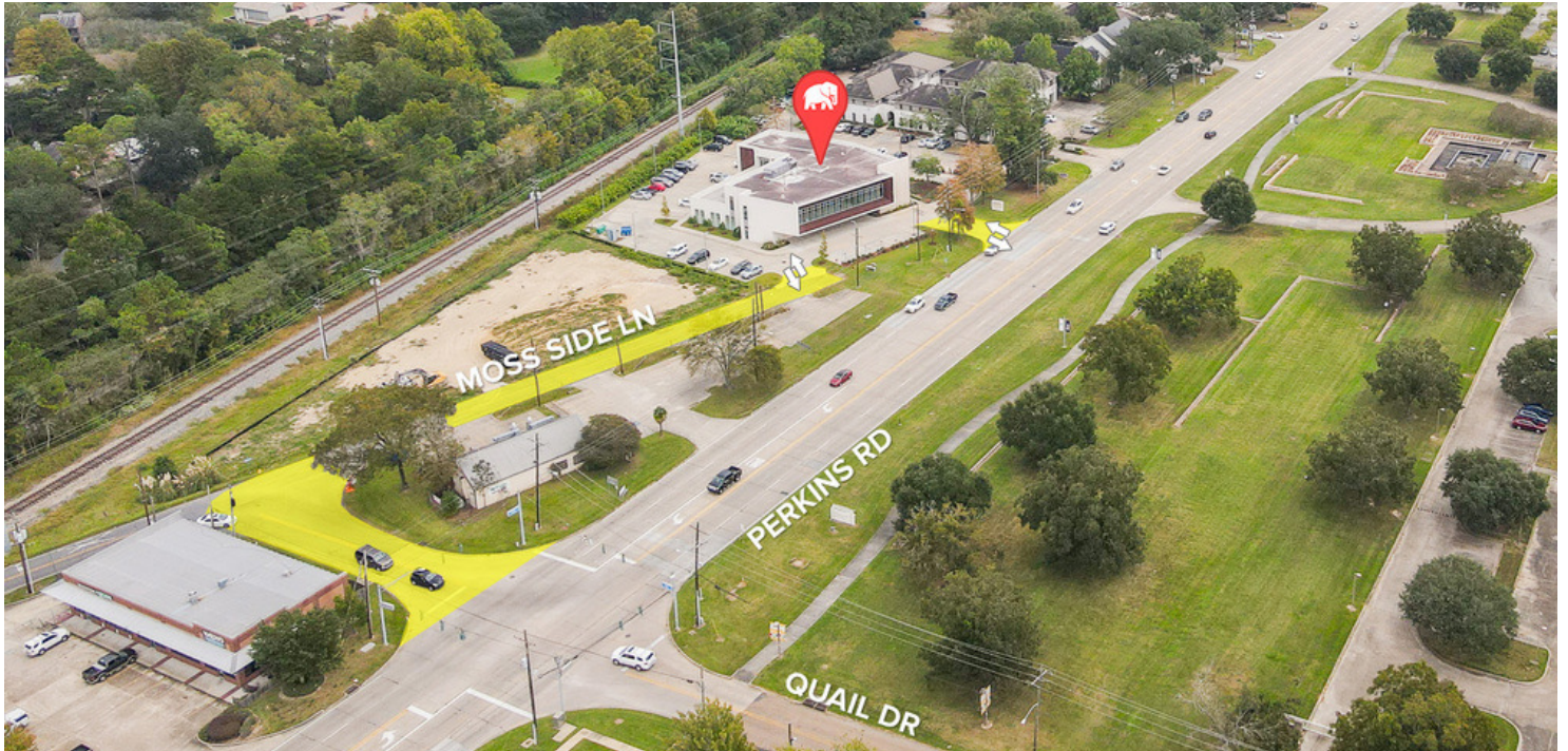
Access points from Perkins Road and Moss Side Lane
