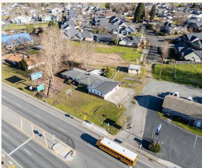
OVERHEAD • THE STRUCTURE, APRON AND HIGHWAY EDGE AT THE SOUTH BOUNDARY
