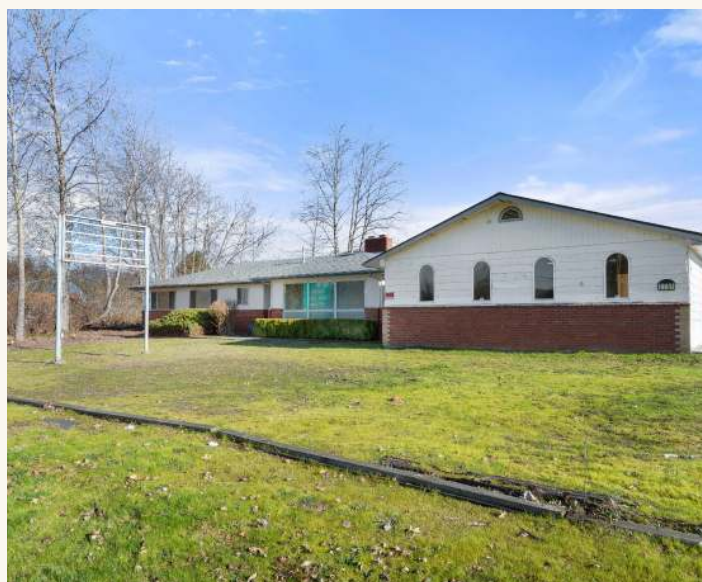
THE EXISTING STRUCTURE FROM THE WILLIAMS HWY FRONTAGE • SINGLE LEVEL, 1958, VACANT
