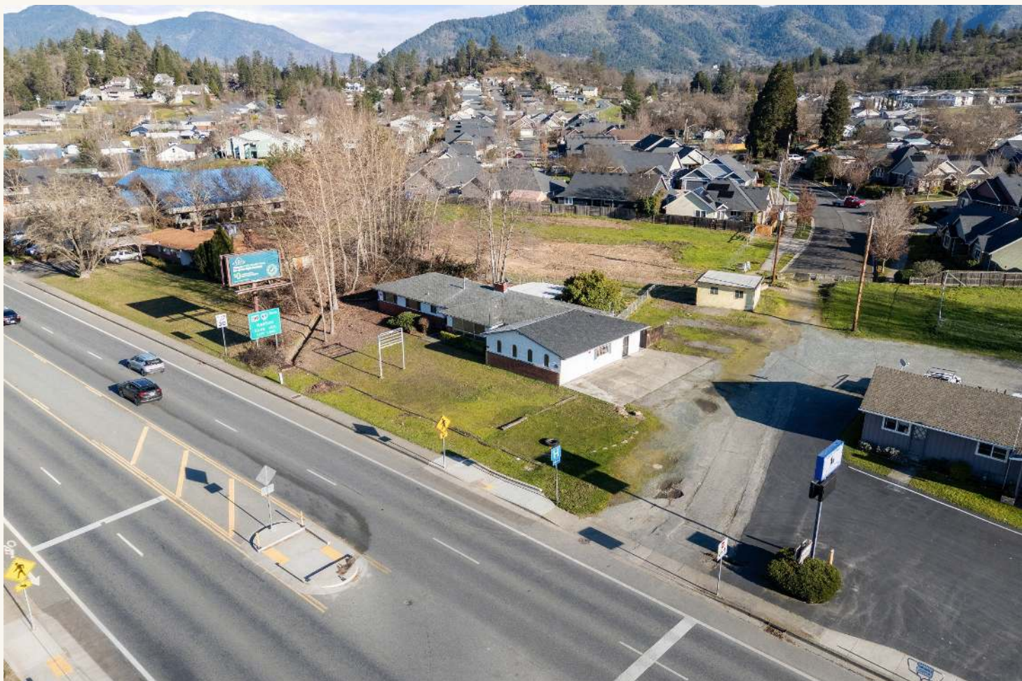
THE FRONTAGE FROM OR-238 • THE GRANDVIEW INTERSECTION AND THE RESIDENTIAL GRID BEHIND
