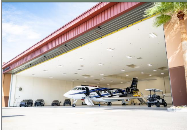
Harry Reid Airport | Las Vegas, NV 26-hangar, 315k SF hangar facility
