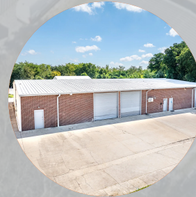
Drive-In doors on front and back of space
