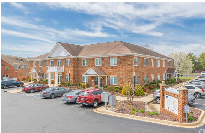
EXTERIOR · EAST ELEVATION
