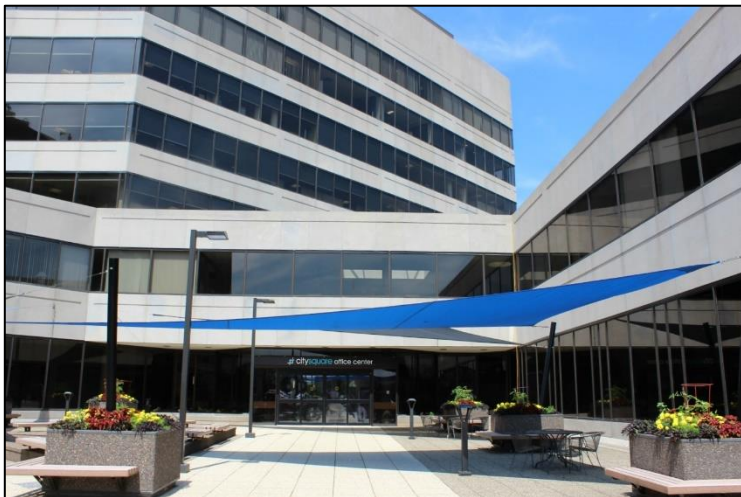
Main Building Entrance (Floor 2)
