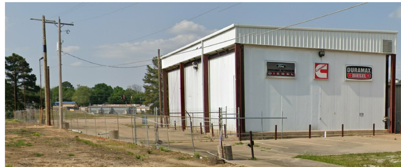
EXISTING STREET VIEW
