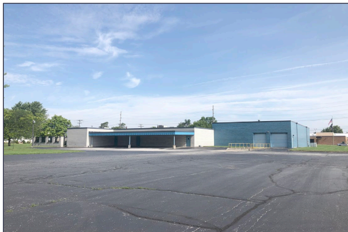
Main Building - Rear view
