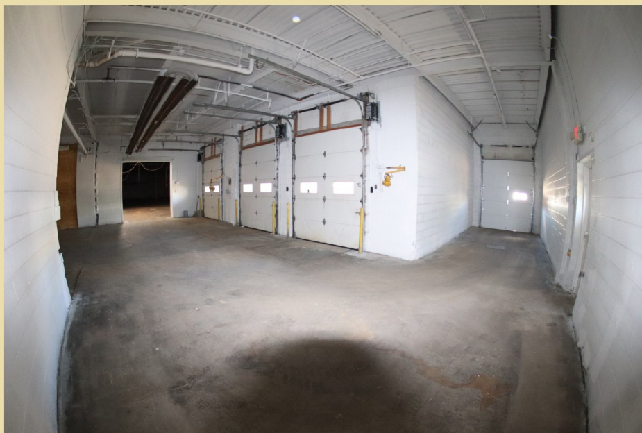
Interior Docks & Drive-In Door
