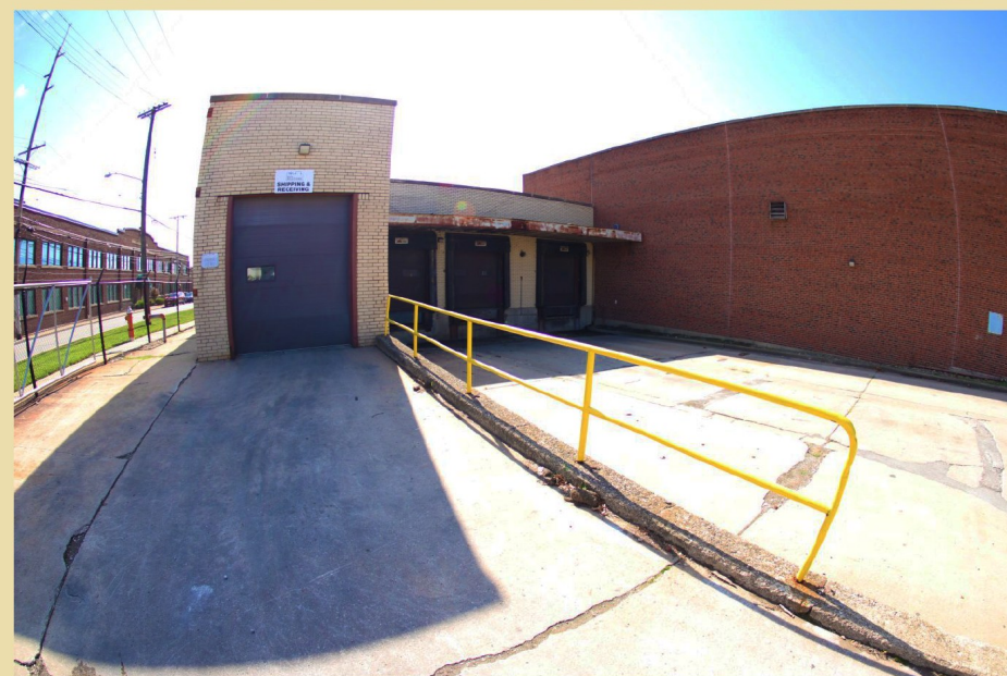
Exterior Docks & Drive-In Door
