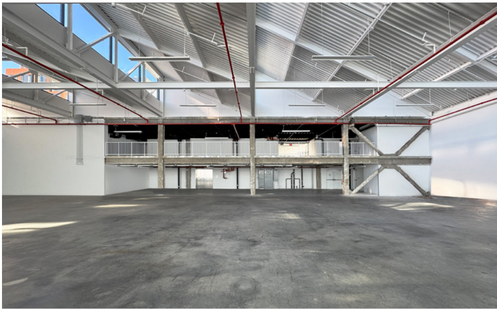
Unit 8 - View of the Mezzanine
