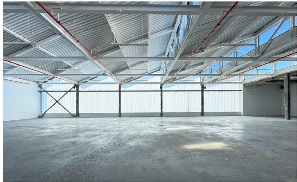
Unit 8 - View of the Translucent Channel Glass Wall
