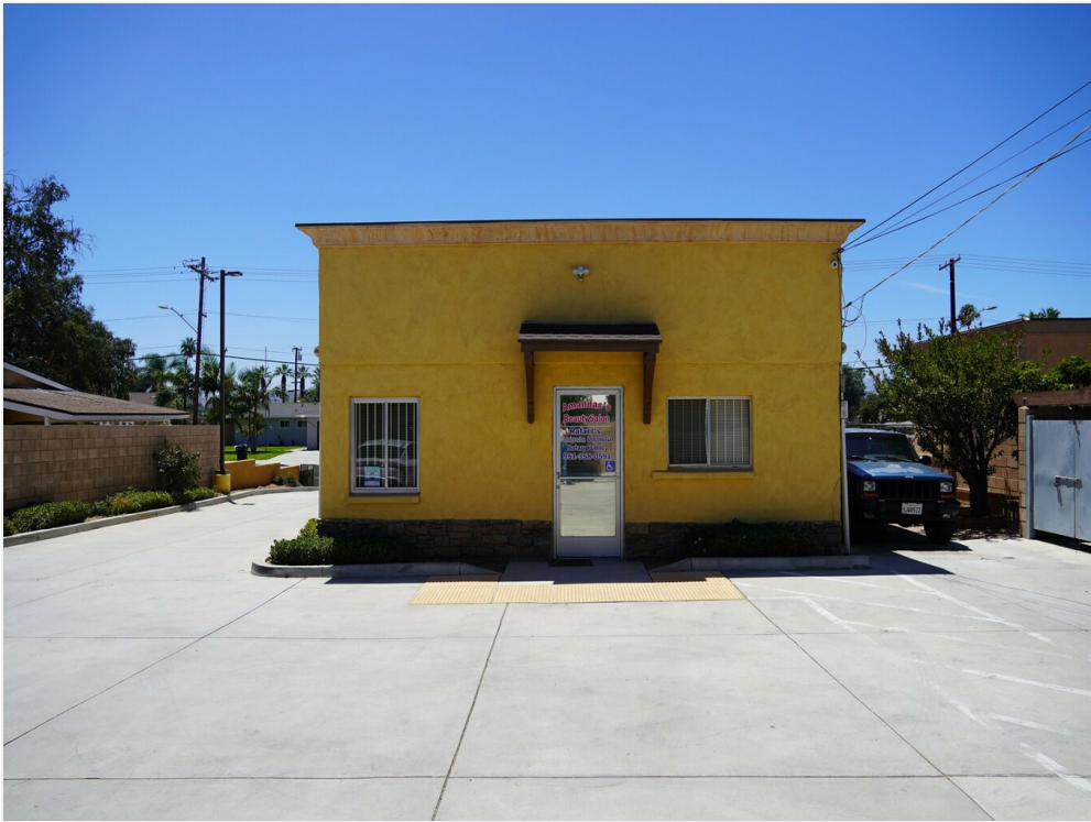
Rear of Building
