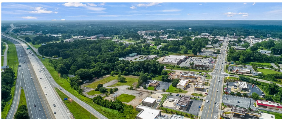
Aerial view along I-75 at the Russell Parkway interchange (Exit 187), Forsyth, GA.
