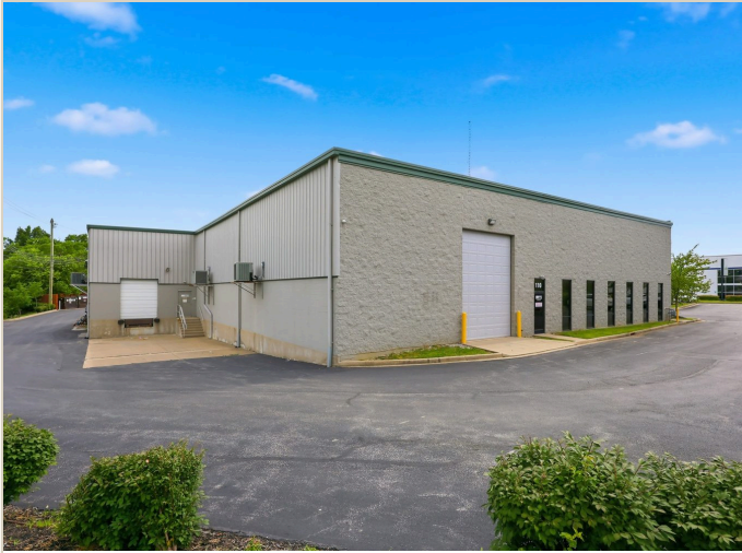
EXTERIOR — DOCK & DRIVE-IN APPROACH
