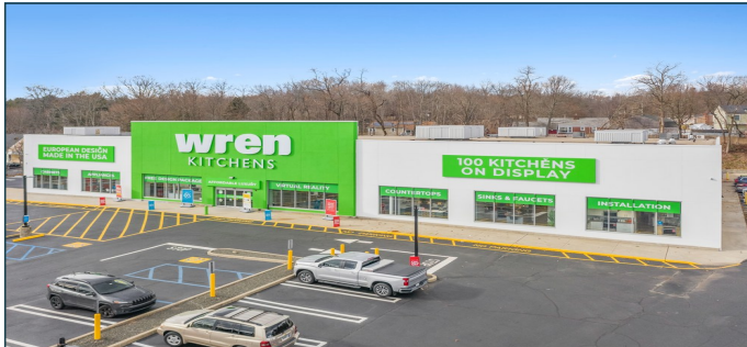
Front Facade & Main Entrance
