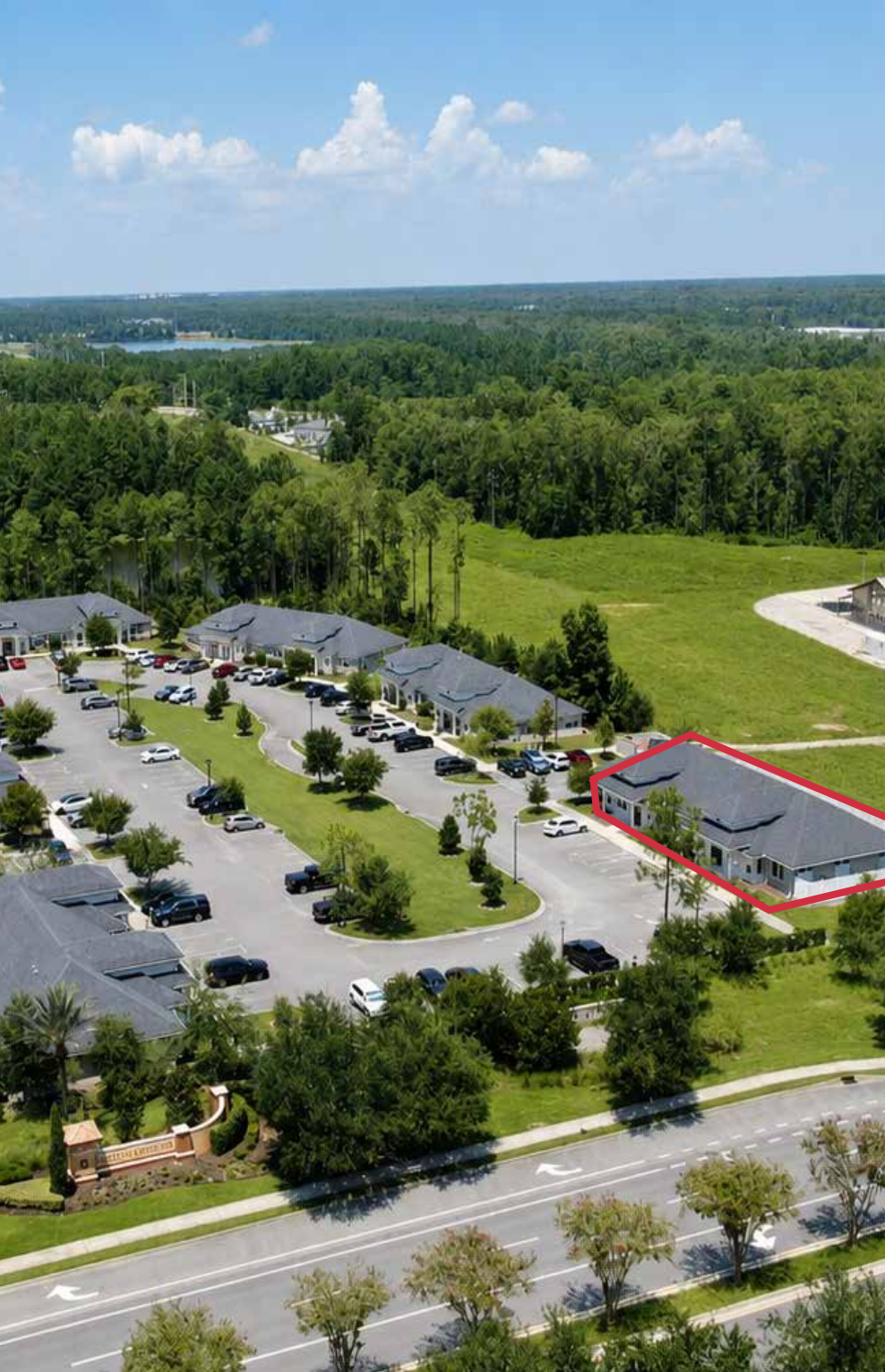
105 DURBIN STATION CT BLDG 400, SAINT JOHNS, FL
