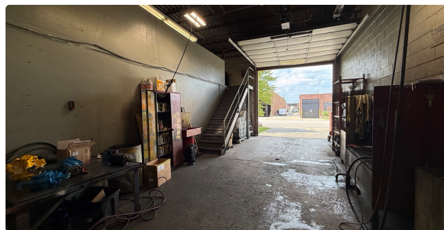
12' drive-in door from inside
