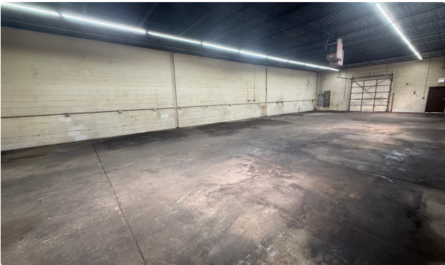
Toward the 10' rear drive-in door
